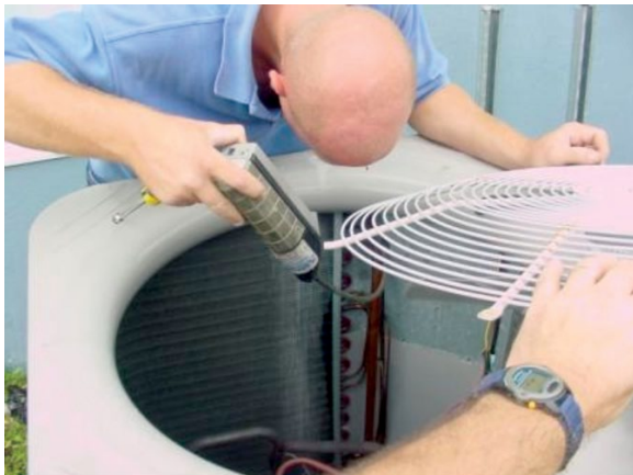
Service technician using sensor to locate refrigerant leak around condenser coil.
